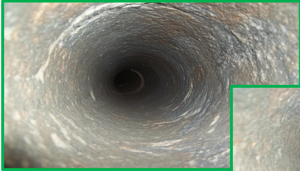
Bitumen liner being removed
