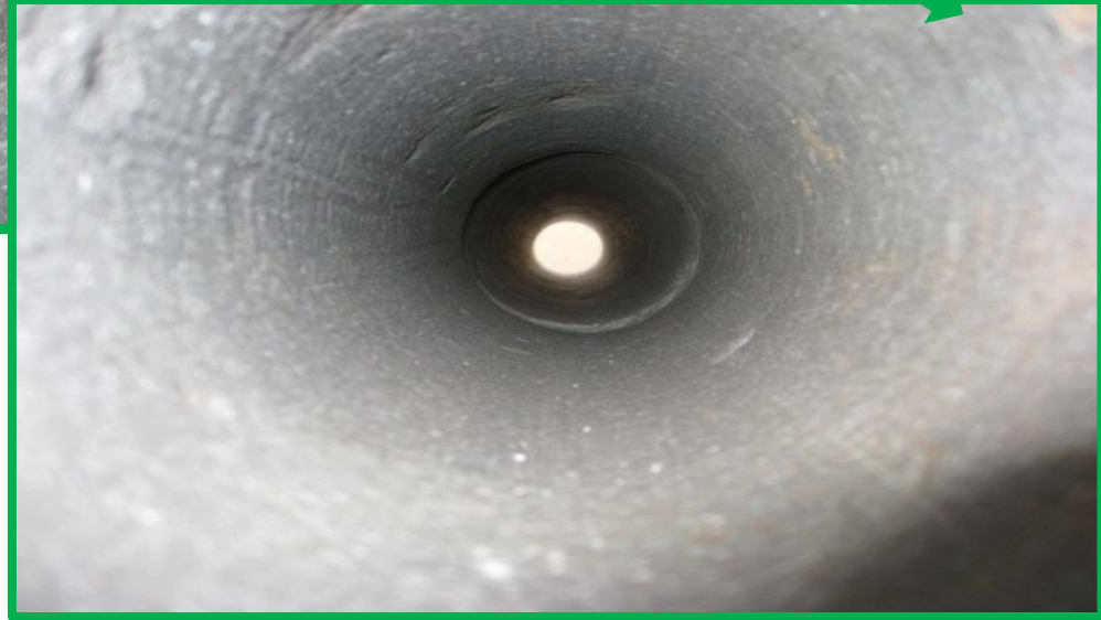
Fully prepared for liner bonding
